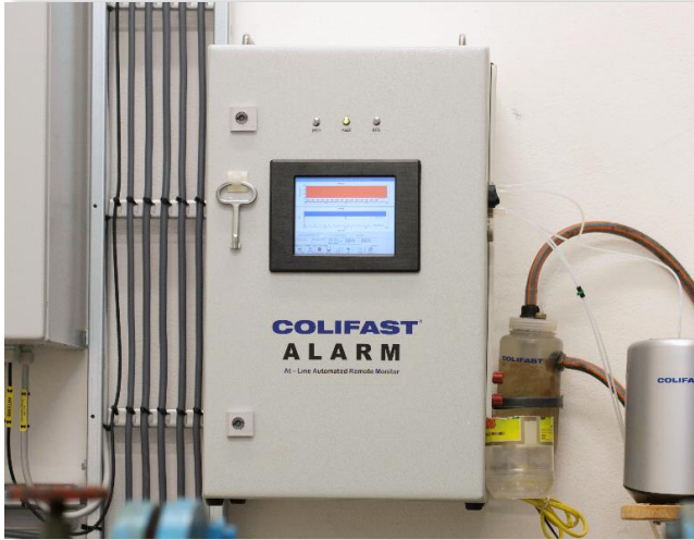
Colifast ALARM at IVAR IKS, monitoring water that is distributed to one of largest food industry areas in Norway.
